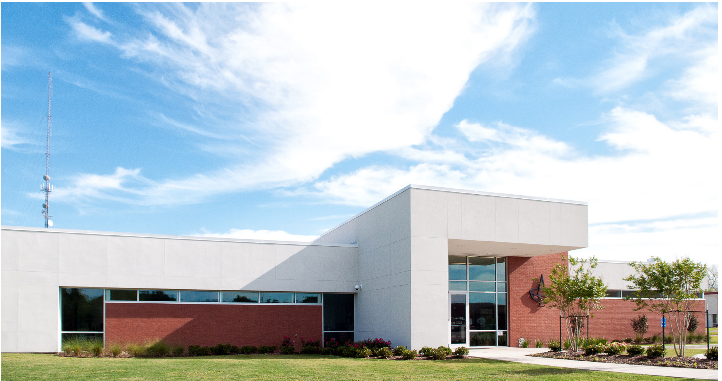
MAIN ENTRANCE © ABM
