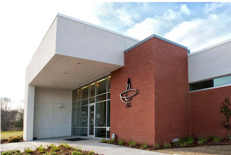
MAIN ENTRANCE CANOPY © ABM
